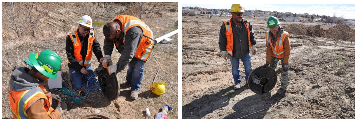
Figure 9 Installation of SmartCover System at Manhole 27
