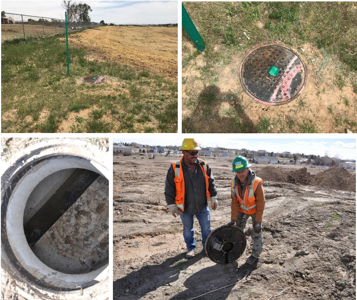
Figure 10 Installation SmartCover System at MH-24
